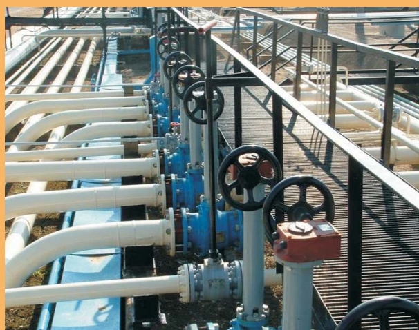
Klinger Ballostar KHI ball valves with flange connection. The gear is attached onto an operating stem extension
