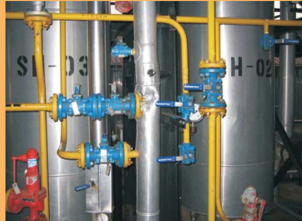
Klinger Ballostar KHA and KHE ball valves with flange connection, manually operated
