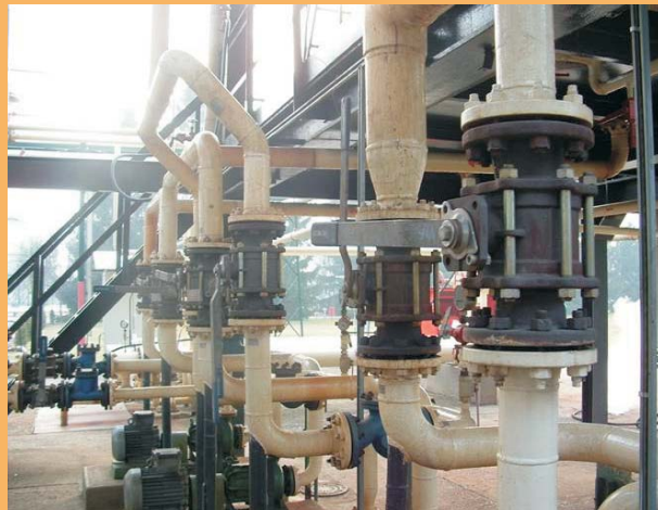
Hand lever operated Klinger Ballostar KHA ball valves with flange connection
