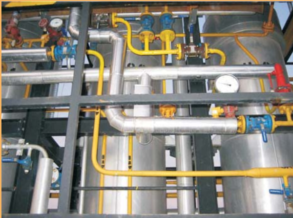
Klinger Ballostar KHA ball valves with flange connection, manual and automated by electro-mechanical actuators
