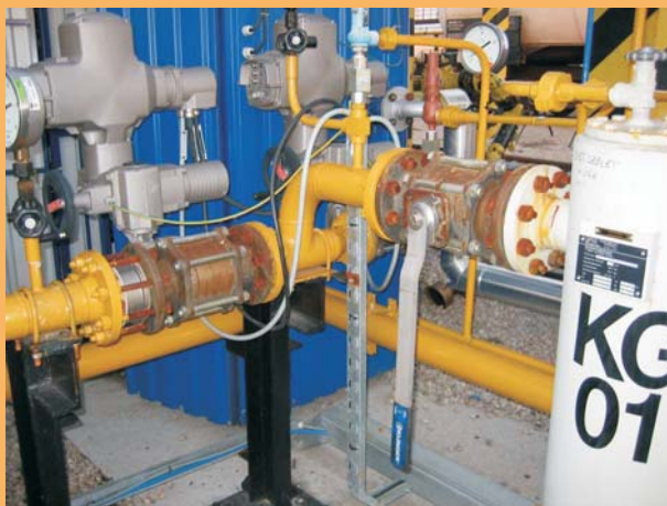
Klinger Ballostar KHA ball valves with flange connection, manual and automated by electro-mechanical actuators
