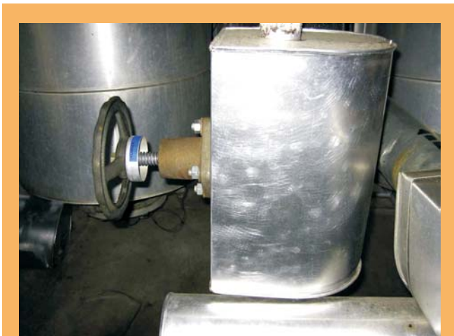
Klinger KVN DN 50 piston valve made of steel casting, fully insulated
