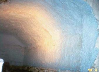
The installation thickness of Foamfrax High Temperature Insulation was maintained at 3" (76mm) across all the lining irregularities of the furnace - so as to not exceed the 3" (76mm) maximum recommended thickness for veneers. The improved consistency of the refractory lining after the installation of Foamfrax High Temperature Insulation provides balanced heating of the charge and results in higher quality forgings.
