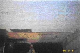
Prior to the installation of Foamfrax High Temperature Insulation, all loose material was removed from the existing refractory ceramic fiber module hotface surfaces. Fiberfrax® Fiberstick <sup>TM</sup> refractory cement was diluted at a ratio of 2:1 Fiberstick to water (by volume) and sprayed onto the existing refractory ceramic fiber module surface. Foamfrax High Temperature Insulation was then gunned directly onto the existing module lining.
