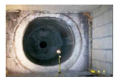
Ductwork transferring hot gas exhaust from a gas turbine to a heat recovery steam generator (HRSG) required high temperature insulation to decrease the cold face temperature and increase thermal efficiency. Gas turbine exit gas velocities decrease in the ductwork section due to increased cross sectional area, and refractory ceramic fiber high temperature insulation is suitable for this application\*.
